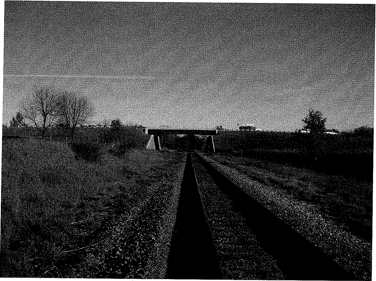
New 57 th Street Overpass
