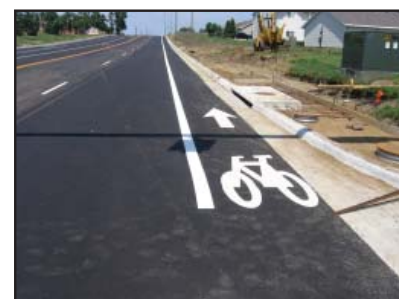
Gutter slope matches the roadway slope to provide an effective 6' wide bike lane along both sides of Sertoma Avenue
