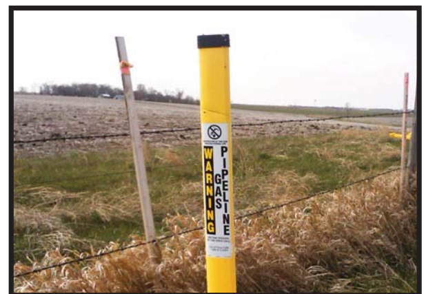
Landfill Gas Pipeline Marker
