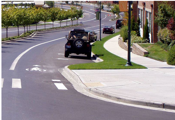
Painted Crosswalk, along with curb ramp
