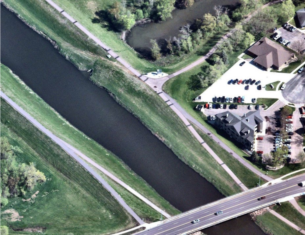
Station Point at Big Sioux River and 49th Street
