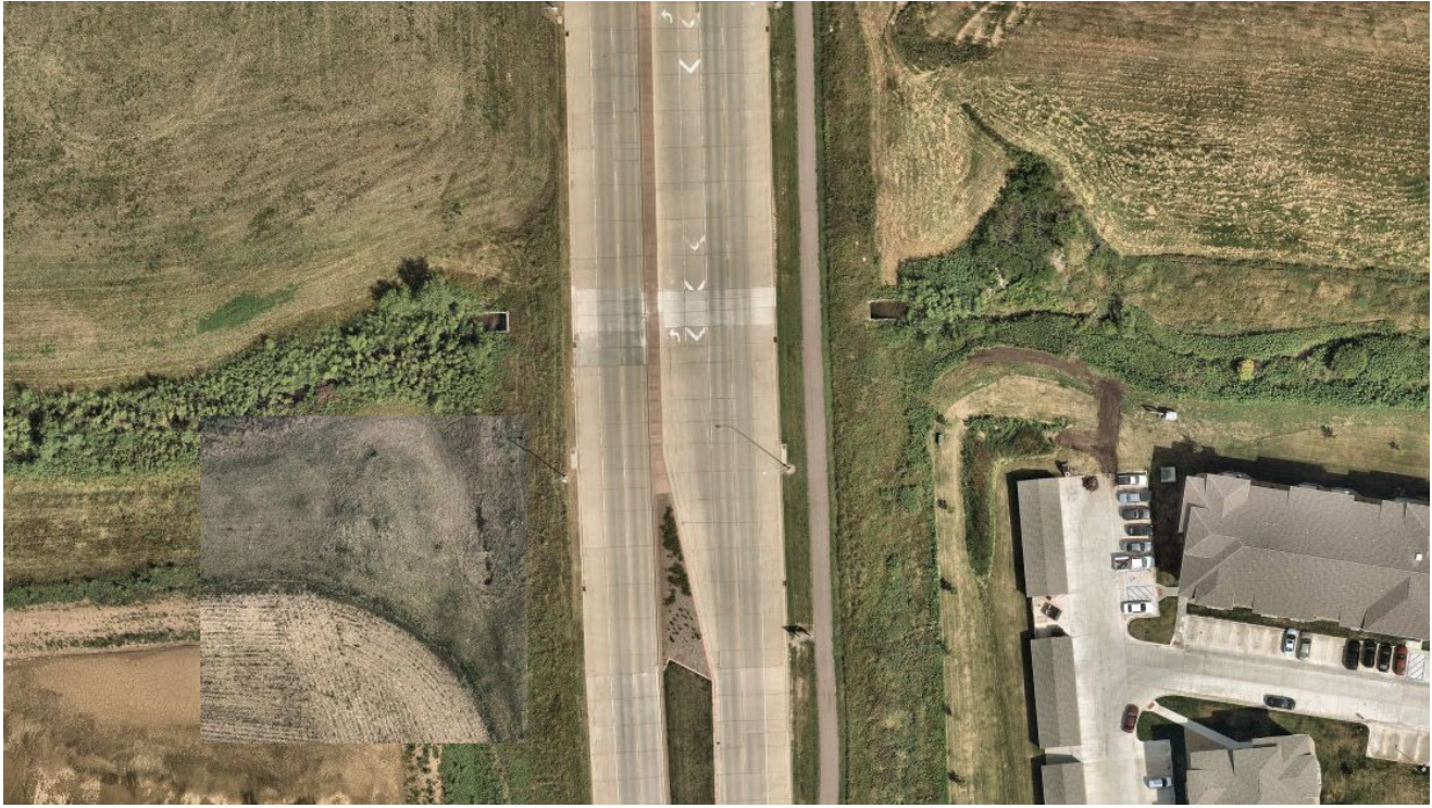
Copper Creek underpass—33rd Street and Veterans Parkway
