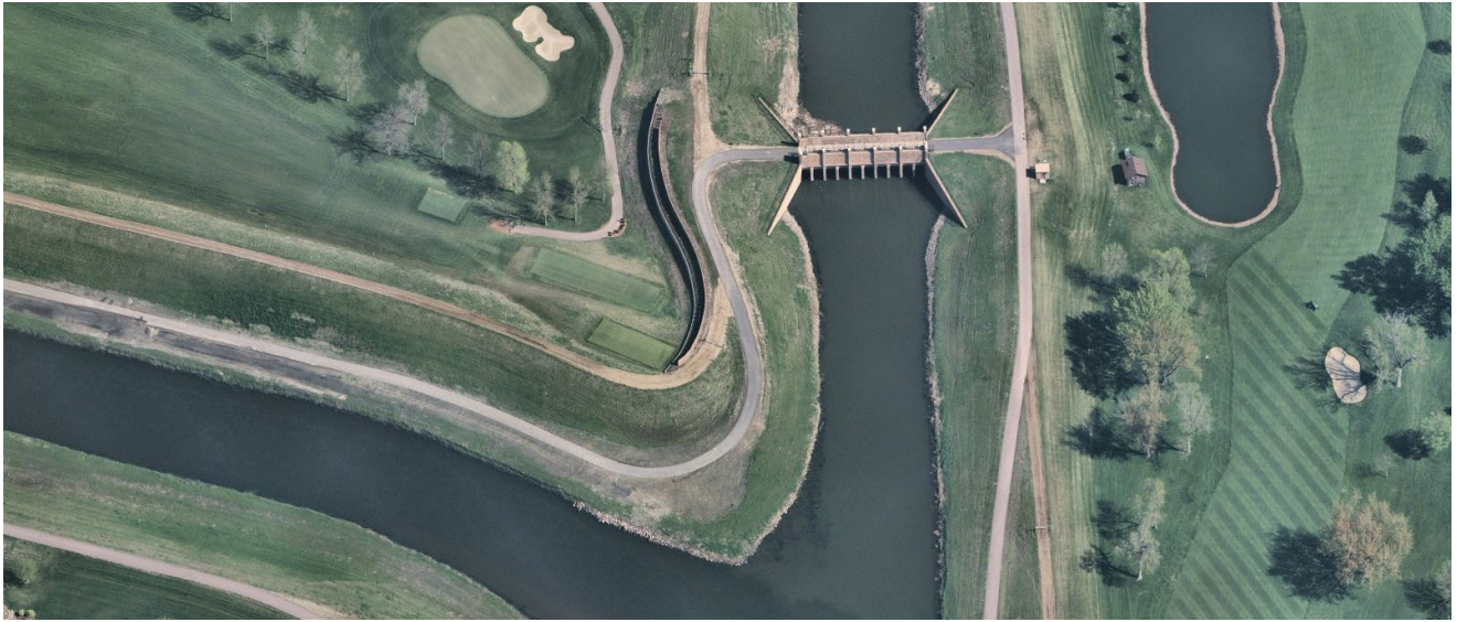
Big Sioux River crossing to west side at Diversion Dam/Golf Course
