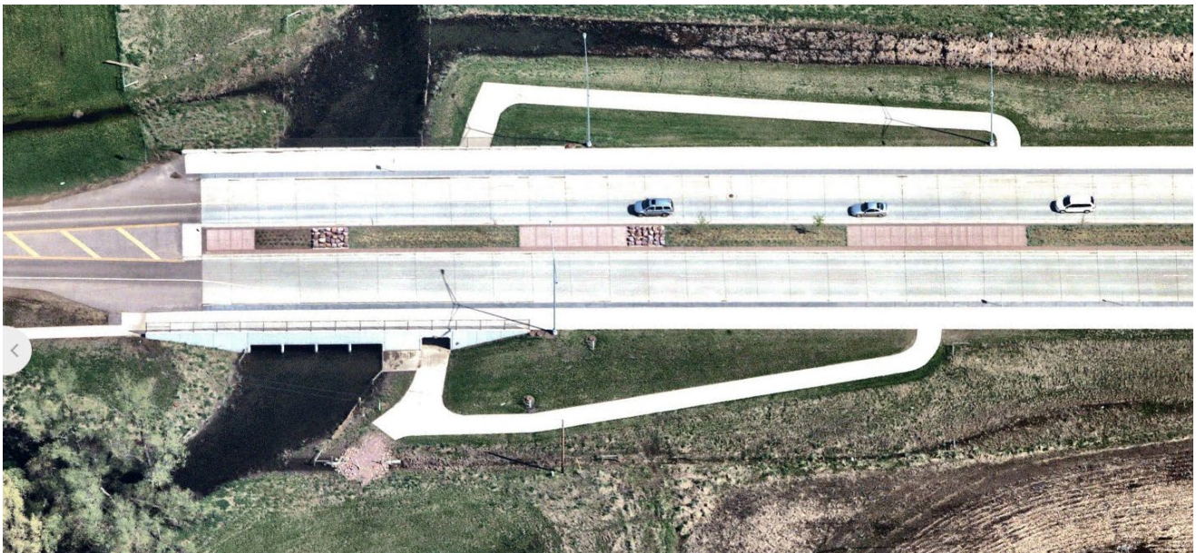
West Maple Street pedestrian underpass west of Marion Road
