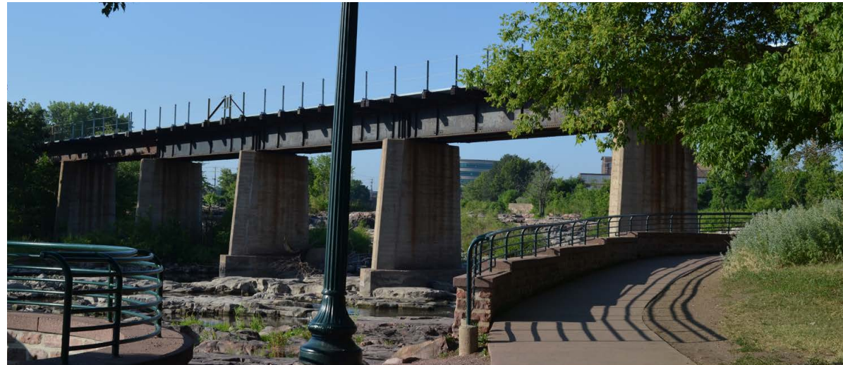
Railroad Bridge and Corridor Through Park
