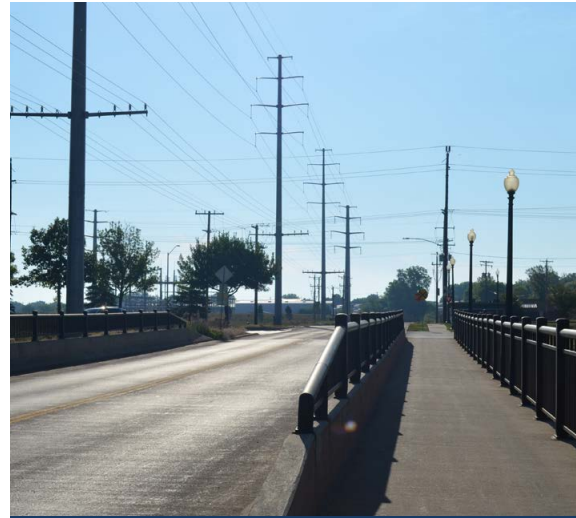
Existing Power Line Corridor Along Falls Park Dr
