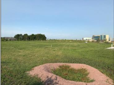
The pictured area had been seeded and is pictured here with good establishment. Having the horseshoe filter in place as pictured was an easy way for this site to remain compliant while waiting for vegetative establishment.
