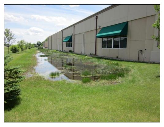
Each rooftop, parking lot, and street collects pollutants. These pollutants are washed away with every rainstorm and end up in downstream water bodies if they do not filter through a BMP. All BMP filters eventually need routine inspection and maintenance to properly function. An improperly maintained BMP results in poor water quality discharge and unwanted flooding to the surrounding infrastructure, much like what is pictured above.
