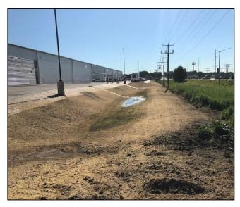
Proper hydro-mulch coverage in conjunction with good erosion control blanket installation helped to drastically reduce erosion on the pictured slope.
