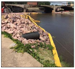
A temporary access road was constructed and the slope was reinforced with large riprap, curtailing the possibility of erosion. Adding silt curtain as pictured helped to further contain any particulates.
