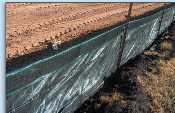
Proper installation of silt fence to protect disturbed soils.
