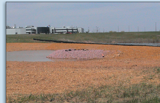
Proper installation of sediment basin, silt fence and seeding/mulching.
