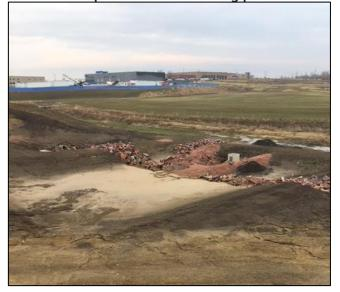
Two building sites on W 54<sup>th</sup> ST N shared a well-built sediment basin. The picture shows how effectively a well-built sediment basin holds back sediment and other particulates during a storm event.
