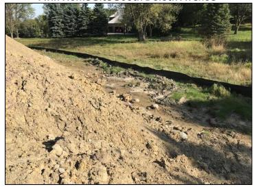
Silt fence and sediment traps in sequence were utilized at this site. One trap upstream of the pictured area helps lessen the load on the far trap and properly installed silt fence.
